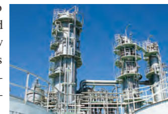
Distillation Plant with complete closed system
