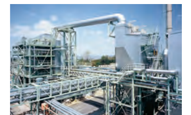
Bio-Mass Power Plant
