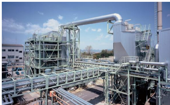
▲Biomass power plant at Kakogawa Site
